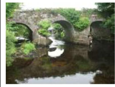
A photograph of the Ardbear Old Bridge, a hump-backed road bridge with three arches, crossing the Owen River. The bridge is built of coursed rubble and features v cut-waters and parapets. The water is calm, reflecting the bridge and the surrounding greenery. |
