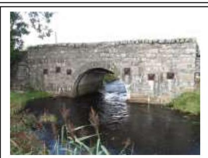
A photograph of a stone bridge with a single arch, crossing a river. The bridge is built with granite rubble and has cast-iron tie-plates.    |
